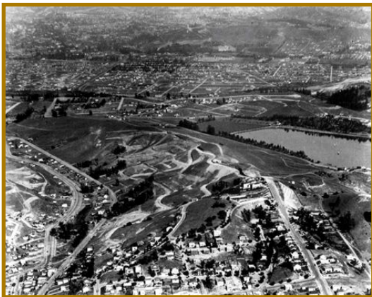
(1930)* - View of the _____ Reservoir named for _____. The reservoir is an earth fill dam, asphalt concrete, with paved slopes. It was put into service in May 1908. In 1989, this reservoir was designated LA Historic-Cultural Monument No. 422.
