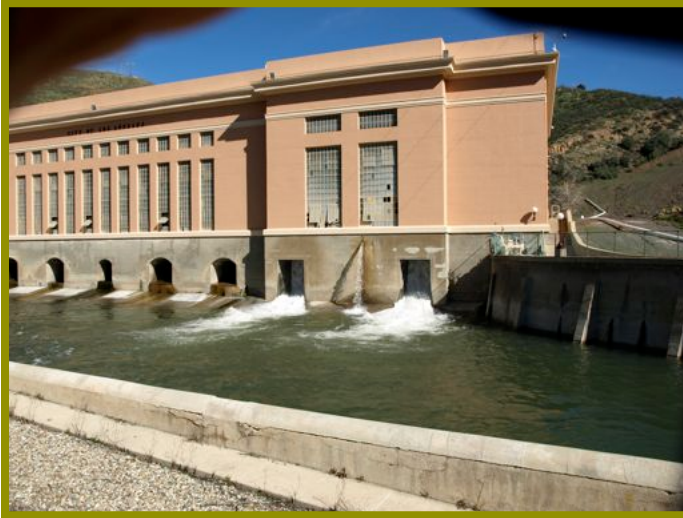
Water exiting the plant going into the tailbay of Power Plant One.
