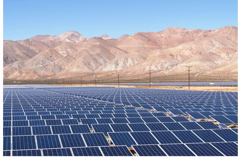
LADWP BEACON SOLAR PROJECT
