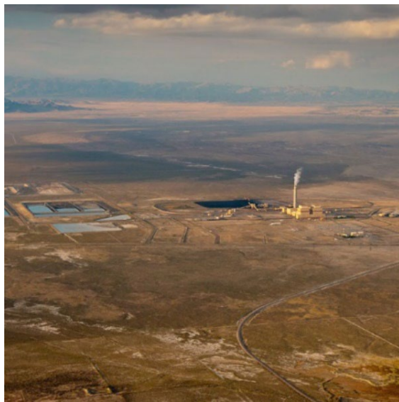
IPP Site Pre-IPP Renewed
