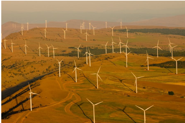
Photo of Windy Point Project, courtesy of Windy Flats Partners, LLC
