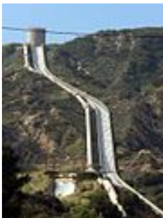
The Terminal Structure and penstock above and alongside the new Cascades on the Los Angeles Aqueduct
