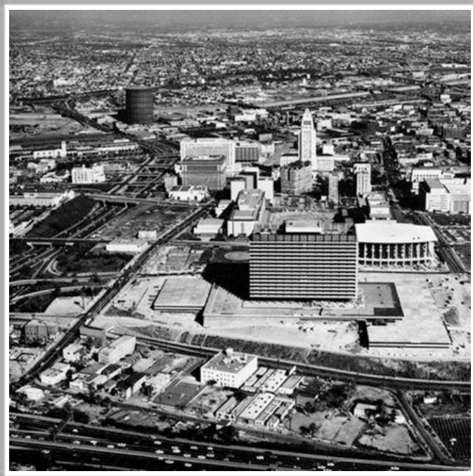
Aerial view looking east toward the Civic Center showing a not quite completed DWP General Office Building (later JFOB) on Bunker Hill.
