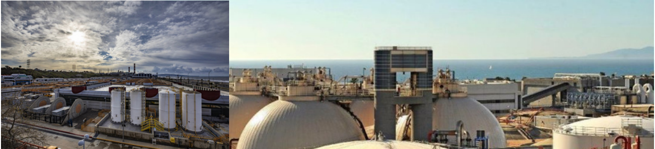
HYPERION TREATMENT PLANT LEFT: LADWP PHOTO; RIGHT: LA TIMES PHOTO
