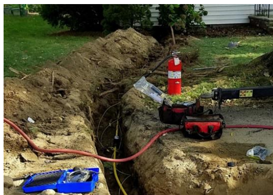
Upgrading a natural gas line in MA
