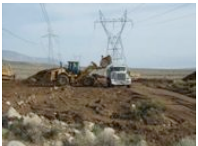
Soil Grading Between Tower 141-5 and Tower 142-1 to Comply with GO 95 Conductor to Ground Clearance Rules
