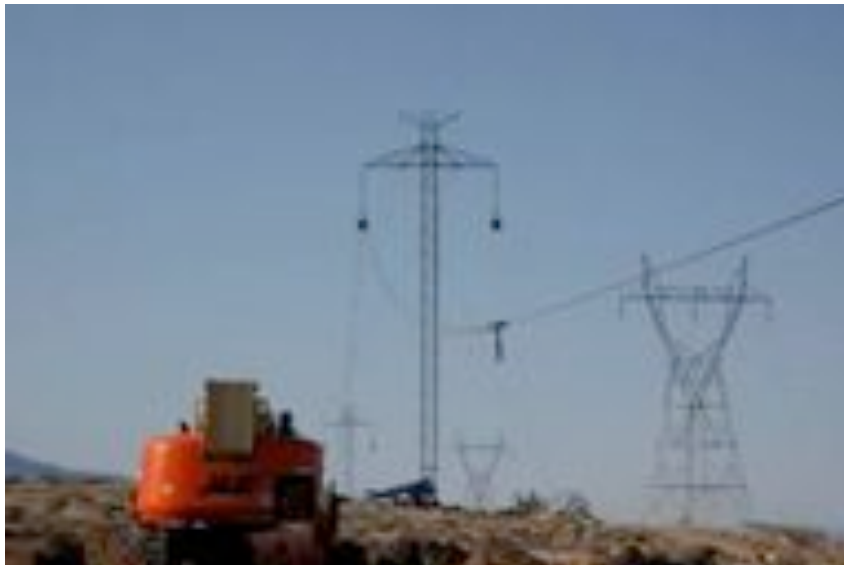
Conductor Stringing
