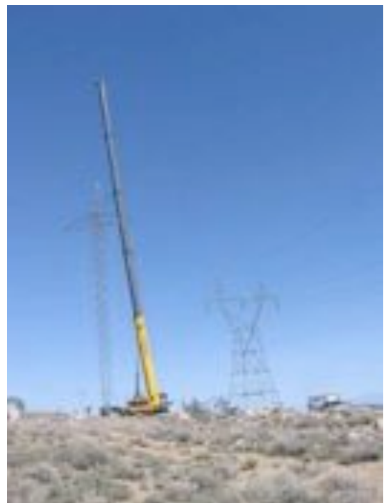
IGS Tower Being Lifted
