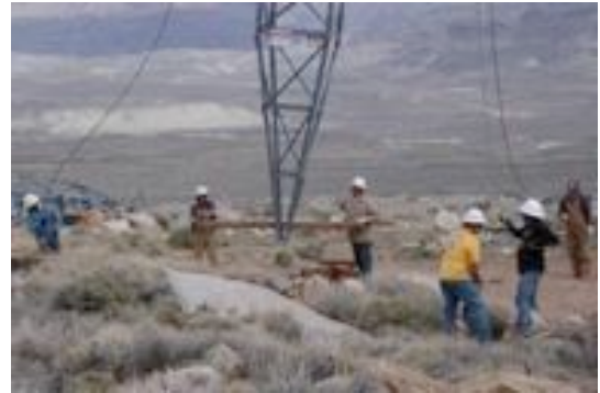
Installation of IGS Tower
