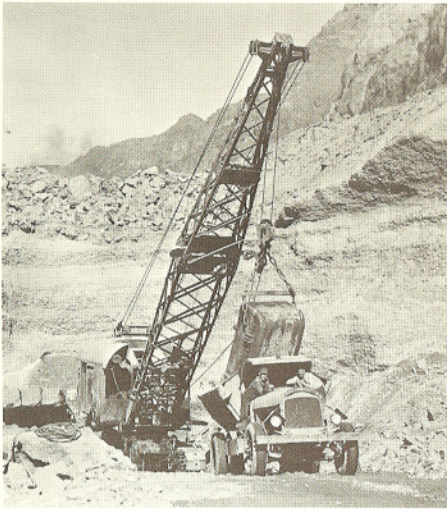
Workmen excavated thousands of tons of riverbed material to reach foundation bedrock for the dam and powerplant.
