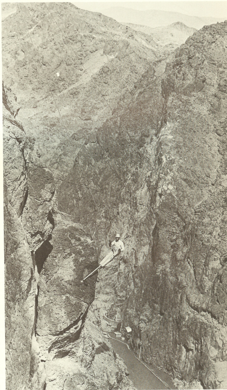
Rigger-rodmen working with topography survey party on Nevada side of Black Canyon at Hoover damsite lowered over canyon rim to provide survey control points which were later used in the design and construction of the dam.
