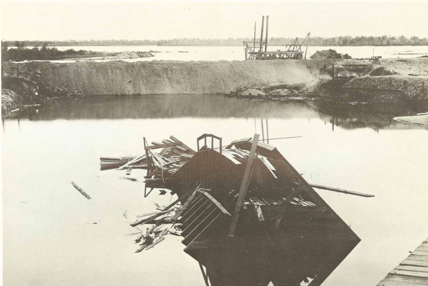
Rock and earth fill barrier was constructed at Imperial Canal inlet after the gates were destroyed in the 1906 flood.
