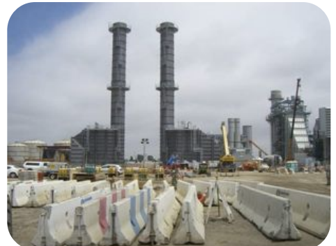
Two of the 100 megawatt gas turbine units.
